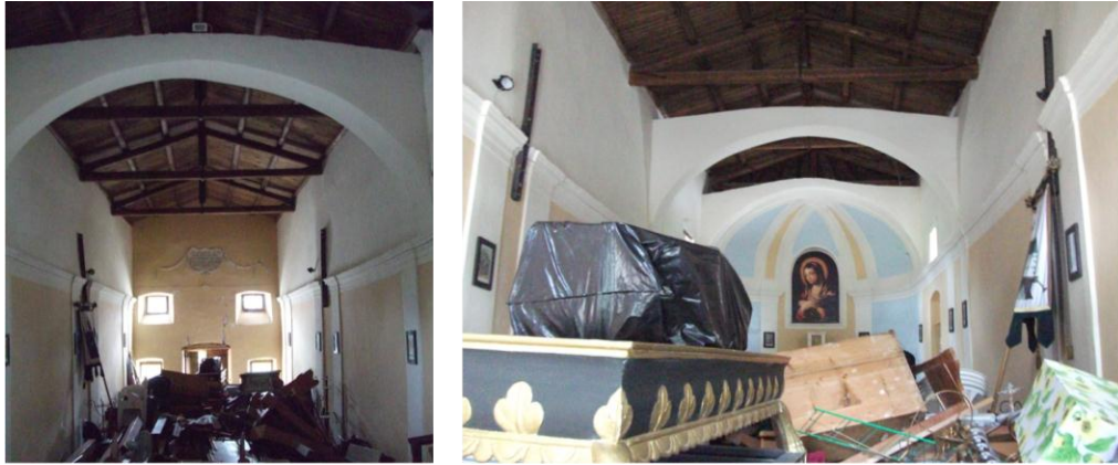
Fig 9. The Visitazione church: internal views
