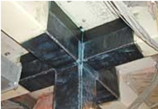
Fig 8. FRP at a beam-column joint
