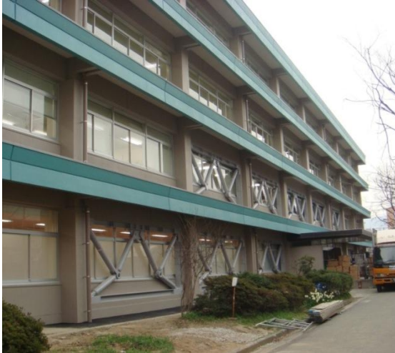
Fig 3. General View of the Building
