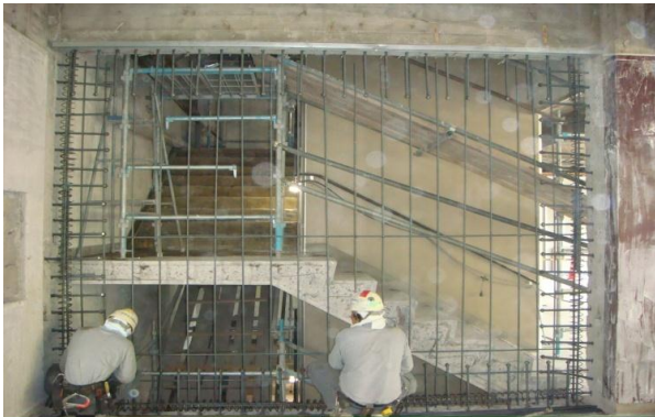
Fig 7. Construction of a shear core
