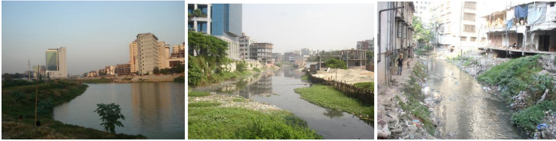
Fig 7. Contemporary Planning with water bodies was never in the development agenda: See the Bagunbari Canal and Kalyanpur canal being encroached indiscriminately.
